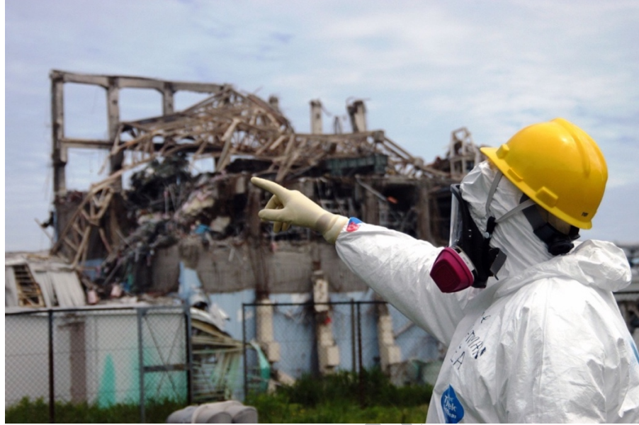
Figure 29: Fukushima Daiichi, Unit 3 after meltdown and hydrogen explosion 245
