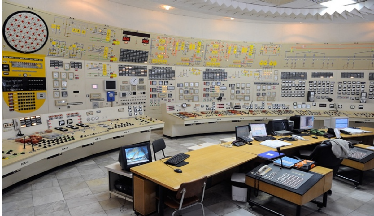
Figure 26: Kozloduy Nuclear Power Plant - Control Room of Units 3 and 4. Control features multiple consuls where data fed from SCADA systems is relayed to control room workers 204
