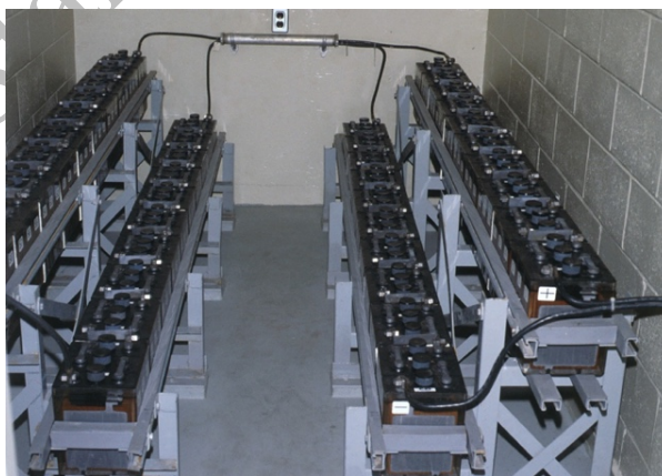
Figure 26: Battery Bank at U.S. Nuclear Power Plant 190
